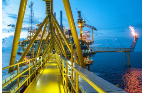
Protection of High-Risk Installations
